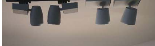
Two of the luminaires above use Luminus Gen 4 COBs and two use conventional 70W metal halide. All four were used in the Light + Building display this year.
